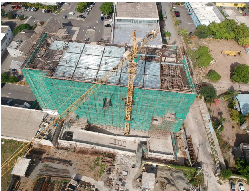
Aerial shot of the new Unit 1 under construction.
