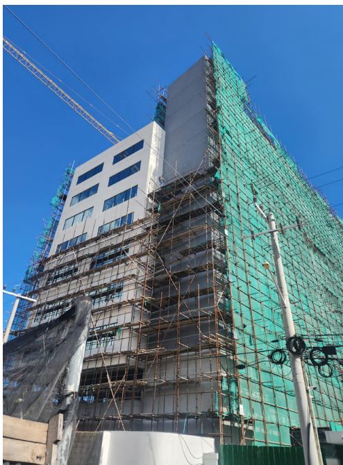
North view of the new Unit 1 best visible from Chelsea Avenue.
