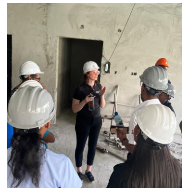
Chairman and CEO, Melanie Subratie leads a group of potential tenants on a tour of the building under construction
