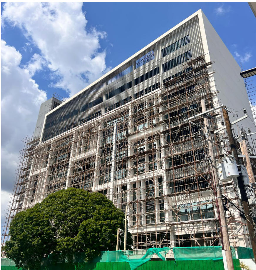
The new Unit 1 is unveiled as the scaffolding is being removed.
