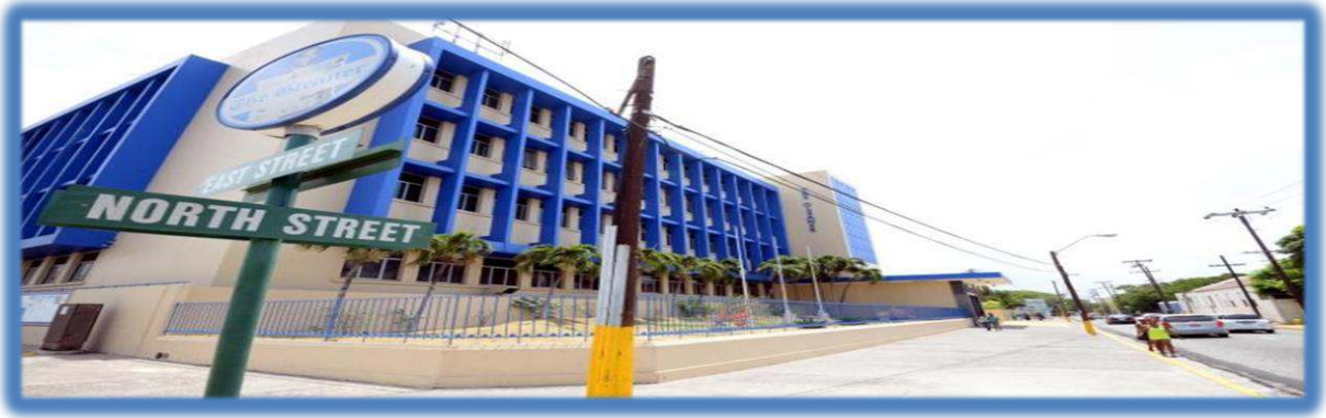
The “Gleaner” Building located at 7 North Street
